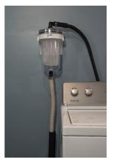
There is a way we can all do our part to reduce the flow of harmful plastics into our lake. I encourage all CCA members to consider installing a microfibre filter on there washing machine. This devise captures microfibres that would otherwise penetrate septic and waste water treatment facilities. Georgian Bay Forev-
